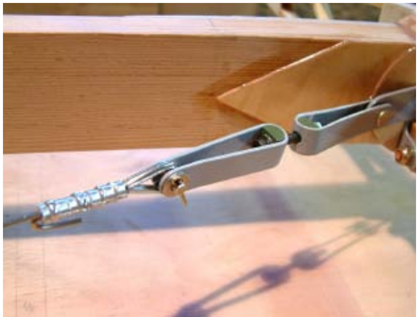
Wing wires are secured with double Nicopress sleeves. The turnbuckles were made at the Flitzer Werke.
