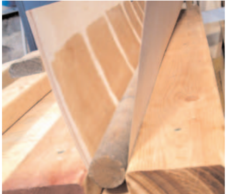
Leading edge plywood was pre-sealed, soaked and pre-bent in this simple tool.
